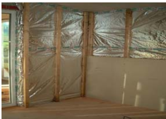
Instalace izolace Lupotherm
