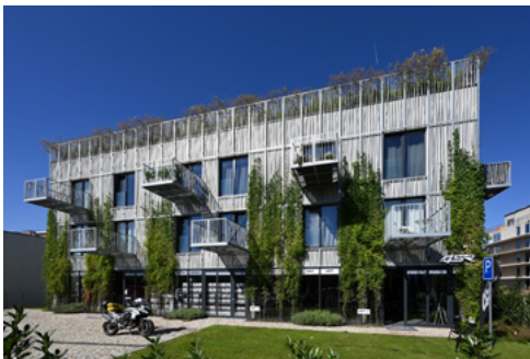
La Vida Residence, Praha / under- construction architects (2022)
